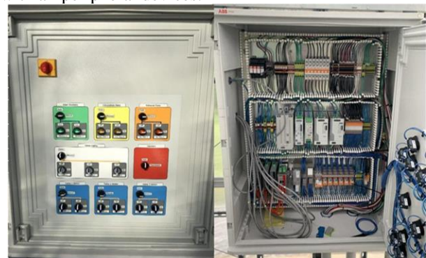
Figure 6. PLC based controller: front panel (left); control circuitry (right)
