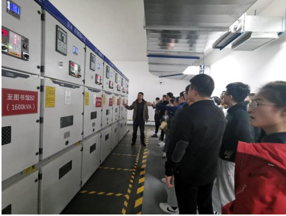
Figure 1. Visiting of campus central substation.
